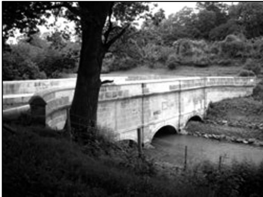
Downstream face of the restored Midford Aqueduct.
