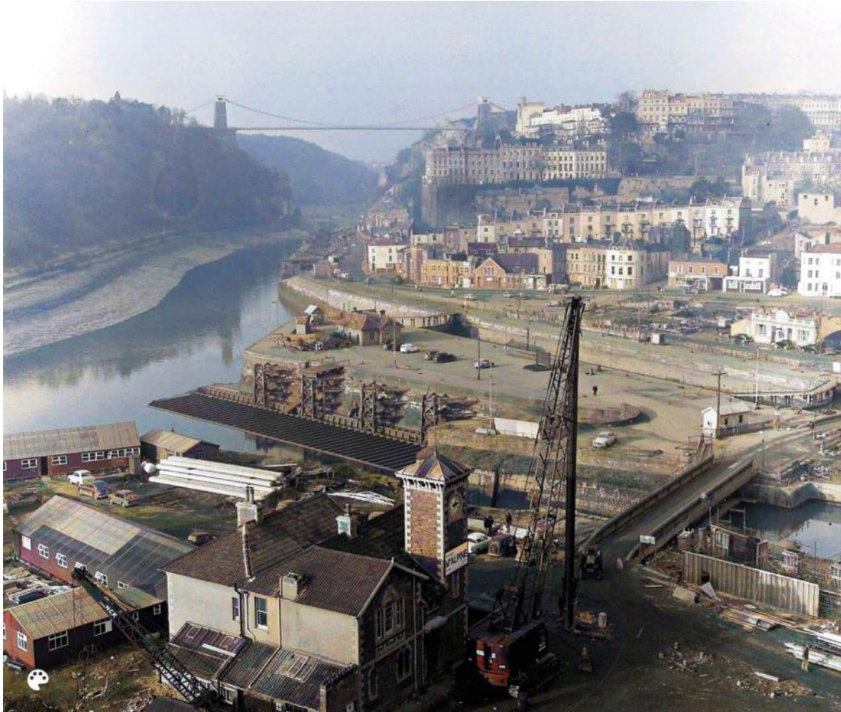
View of the Tongue in 1963 before the Plimsoll Bridge was built. Bristol History Group Facebook Page
