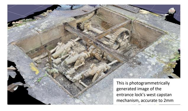
Many of the heritage assets are actually hidden from view in underground pits and manholes or below water (or mud) which makes surveying difficult, so we have to extrapolate known data.
