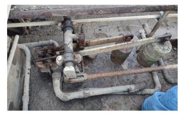
The pressurised water supplied from Underfall Yard was piped to valves beside each jigger. Each valve was operated by a lever slid through a slot in the cast iron cover-plate to lift weighted levers illustrated above. These weights would also have released the pressure if anything went wrong.
