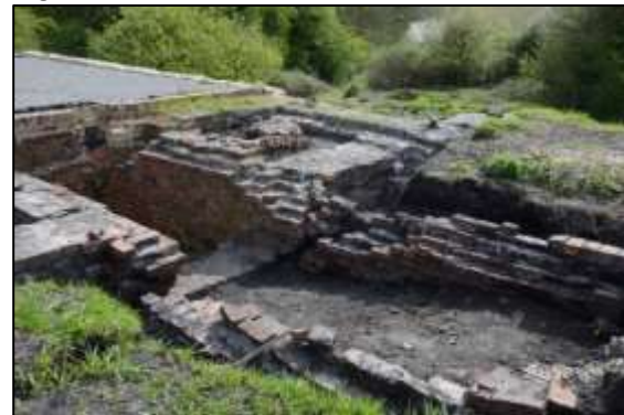
Photo 19 – ... View of the ramp in April 2017 after the walls had been exposed ...
