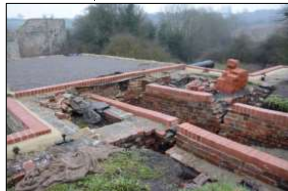
Photo 20 – ... and in January 2018 after the reconstruction.
