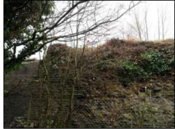
Photo 6 – Vegetation covering the top of the north-western wall of the New Pit heapstead in January 2017.
