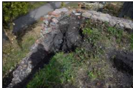
Photo 14 – Close-up of the northern tippler slot, New Pit heapstead, after excavation in April 2017 ...
