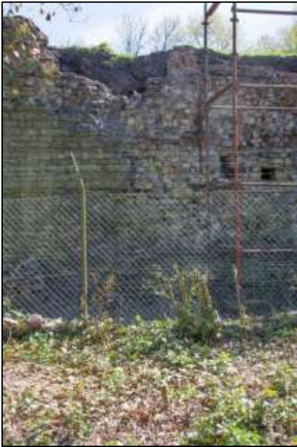
Photo 9 – The north-western wall of the New Pit heapstead in April 2017 after the vegetation had been removed. The break at the top to the left of the scaffolding shows the location of the northern tippler slot.
