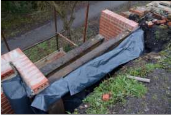
Photo 15 – ... and in January 2018 after the rebuild had been completed.
