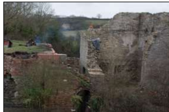
Photo 21 – The rough southern face of the bob wall of the Cornish Engine House can be seen in the centre of this photo, which was taken from the top of the Horizontal Engine House in March 2017 ...
