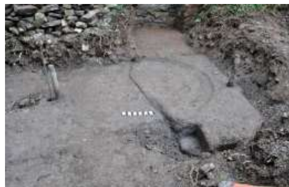
Figure 2 – Engine bed in Cornish Engine House, showing the crack running through the stone base and the annular groove worn into its top surface.
