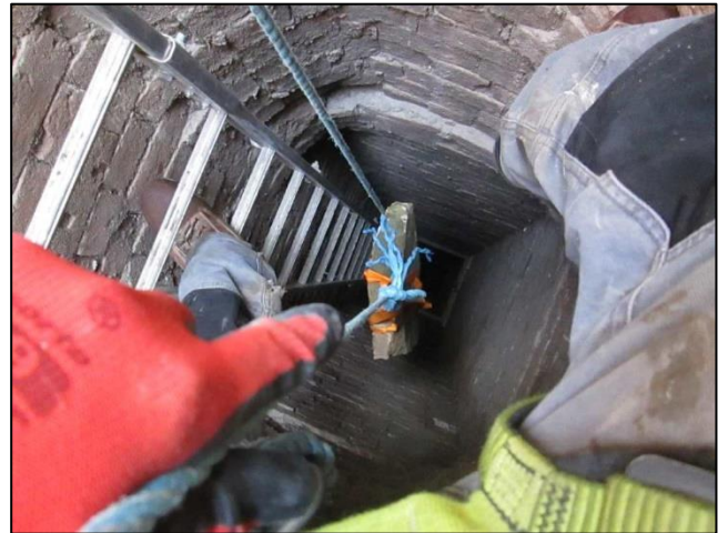
Photo 32 – A replacement stone is hoisted up the inside of the chimney during the rebuilding of the top in 2014. (© C Skelton 2014)
