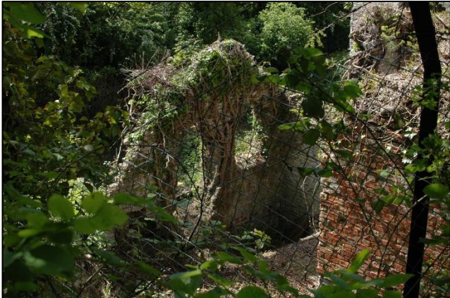
Photo 29 – A view of the Vertical Engine House in 2005, just a few years before the trust started work. It shows that a large part of the south-east wall was still standing at that date. (© M Adams 2005)
