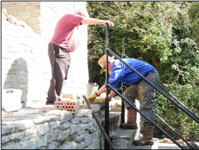
Photo 1 – Jeff and Hamish working on a temporary rebuild at the top of the steps outside the south-west wall of the Cornish Engine House before the HODs.
