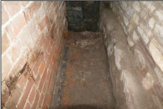
Photo 14 – View along the south-eastern wall of the undercroft with the pit seen in the previous photo at the top of the picture.
