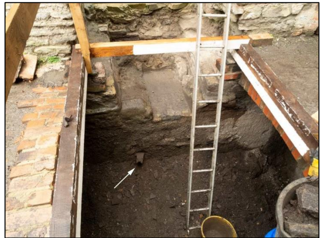
Photo 5 – The position of the pipe clip on the bob wall of the Cornish Engine House has been marked with an arrow. (See comments on p.2)
