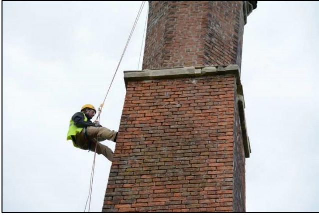
Photo 22 – Charlie working on repointing the outside of the chimney in 2016.
