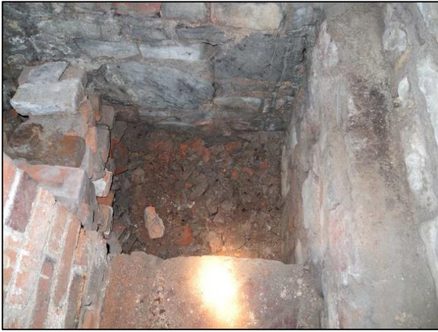
Photo 13 – The pit in the eastern corner of the Horizontal Engine House’s undercroft. (See comments on p.3)
