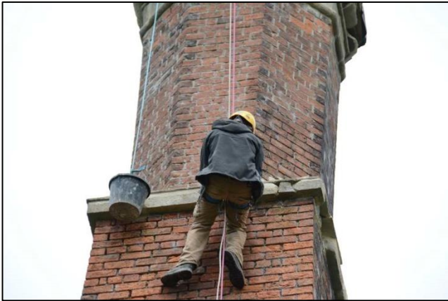
Photo 23 – Charlie working on the shoulder at the top of the square section of the chimney in 2016.
