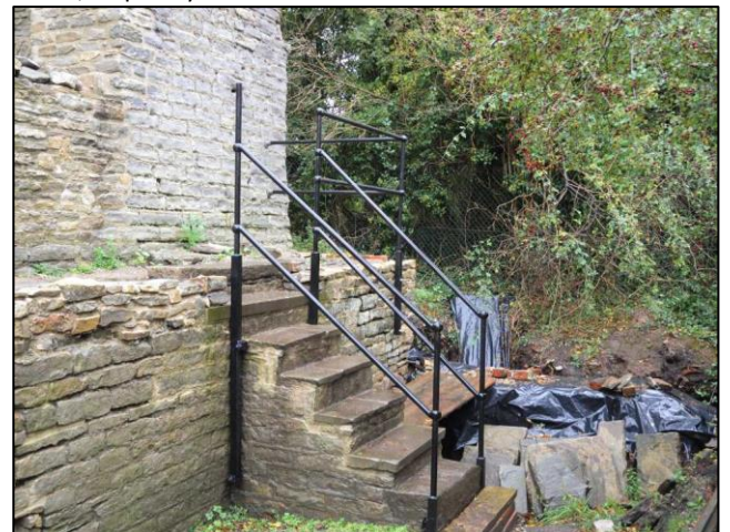
Photo 12 – The completed railings at the south-eastern end of the platform outside the Cornish Engine House at the beginning of November.
