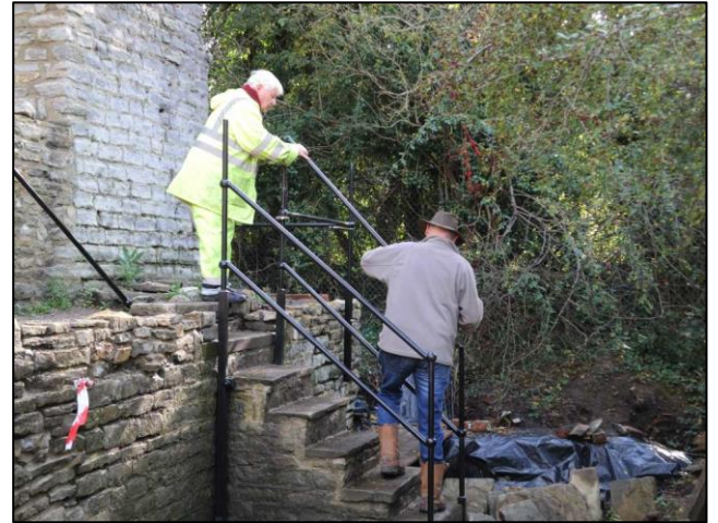
Photo 11 – Jeff working on the railings outside the Cornish Engine House, helped by Hamish.
