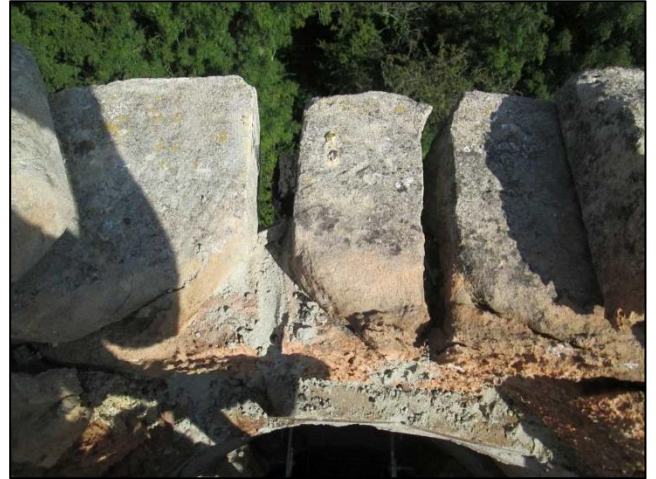
Photo 31 – With the passing of time the mortar had been eroded from between the stones at the top of the chimney, leaving the large gaps seen in the photo. These gaps could be seen from ground level. (© C Skelton 2014)
