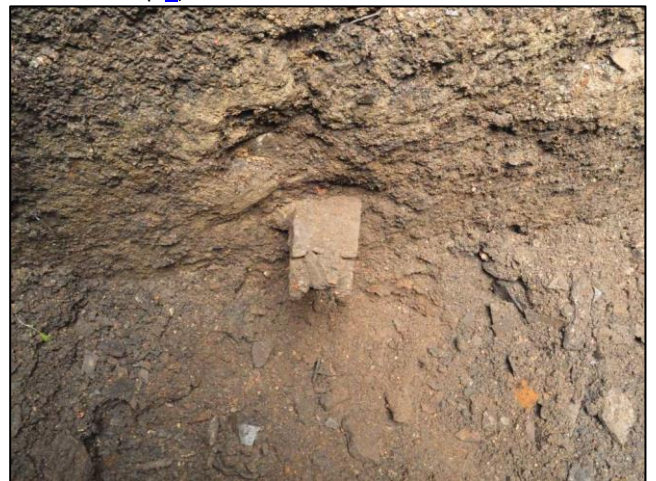
Photo 6 – Close-up of the pipe clip sticking out of the bob wall of the Cornish Engine House before the covering stones were removed.
