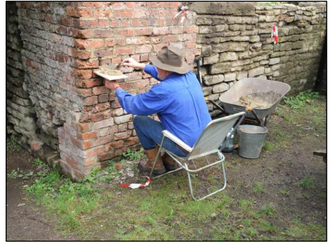
Photo 10 – Hamish takes it easy when repointing the brickwork by the entrance to Pumping Shaft passage.
