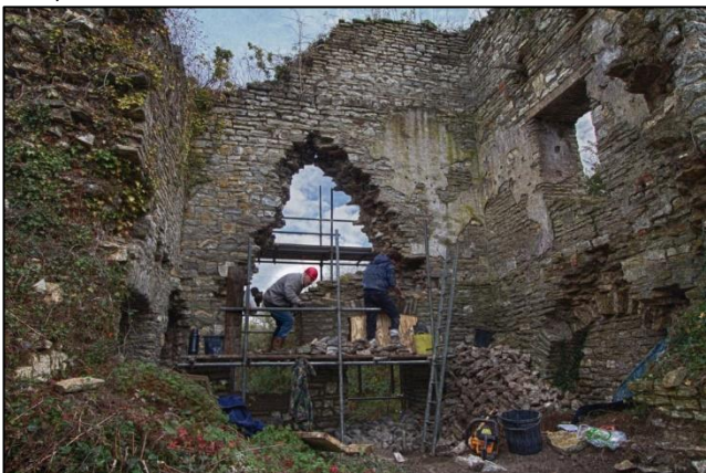
Photo 30 – The inside of the Cornish Engine House during the rebuilding of the north-east wall in 2012. (© M Cole 2012)
