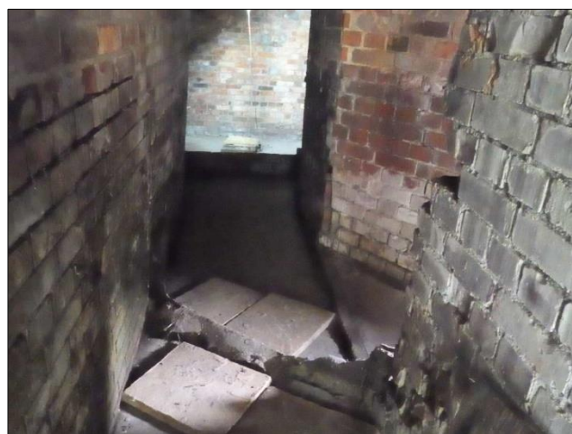
Photo 7 – The inside of the southern fan duct, with the white slabs on the floor protecting the remains of a damper in the foreground. The chamber in the background, which is common to both ducts, was artificially lit so that visitors could look around.
