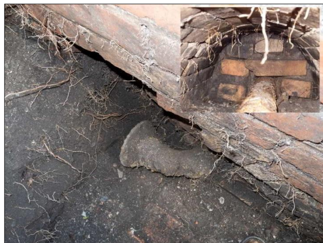
Photo 14 – The outer end of the pipe that runs through the tunnel in the eastern wall of the egg-ended boiler settings. The inset shows the inside of the tunnel and was originally published as photo 14 of Newsletter 34.
