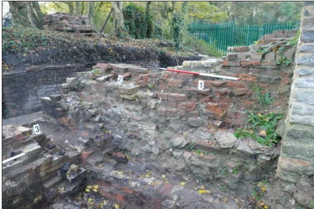
Photo 23 – Exposed brickwork at the north-east end of the Egg-ended Boiler settings in November 2022. (1 m ranging pole)
