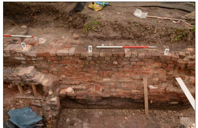
Photo 37 – Part of the south-east wall of the boiler settings. This, and the other photos have yet to be combined into a composite. (1 m ranging pole)
