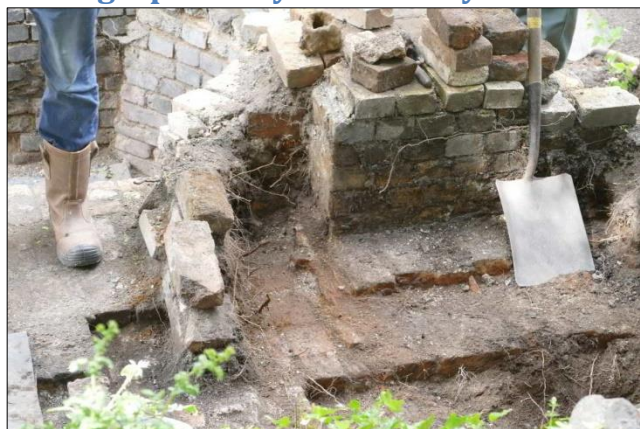
Photo 11 – Close-up of the brickwork at the end of the Egg-ended Boiler settings. A general view of this area can be seen in photo 12 below.
