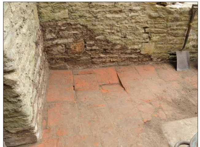
Photo 44 – The sagging floor in the south corner of the Cornish Engine House (See comments on p. 3 ) ...
