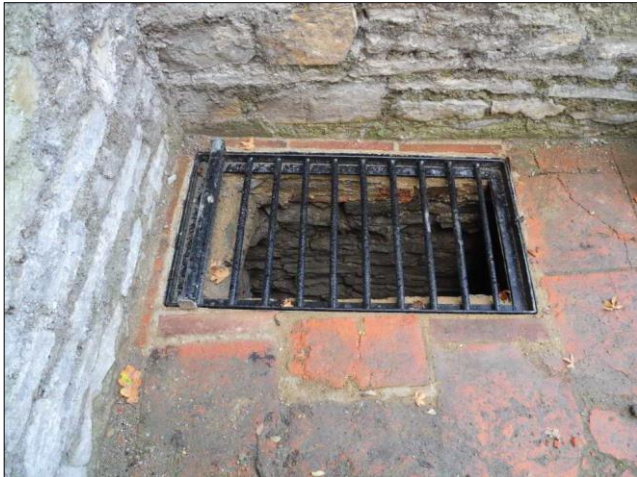
Photo 46 – ... A permanent metal grille has been fitted to the hole.
