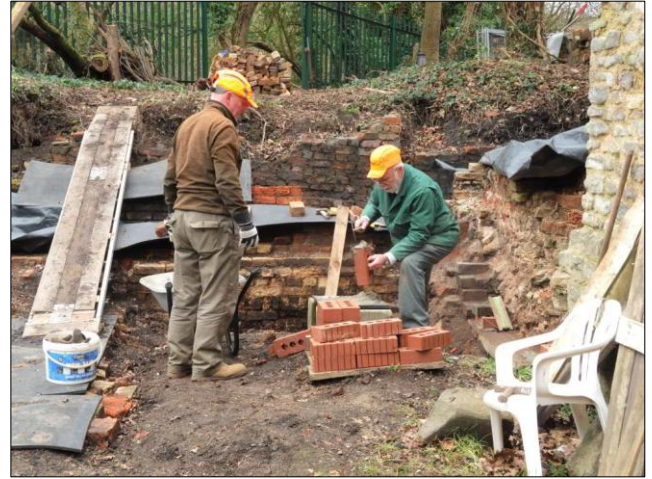
Photo 24 – John learns the art of bricklaying from Ken, as they worked on conserving the outer side of the north-east end of the Egg-ended boiler settings ...
