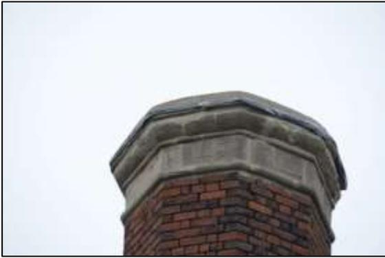
Photo 3 – ...and the top in March 2015 once the masonry section had been repointed.
