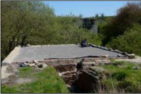
Photo 21 – Trimming the excess waterproof membrane on the roof of the Horizontal Engine House.
