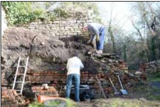
Photo 11 – Clearing the spoil from above the East Flue.
