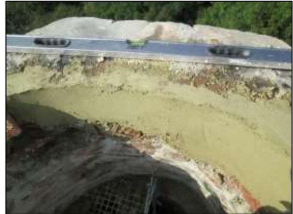
Photo 6 – Making the foundations for the cast concrete ring. © C Skelton, 2014.
