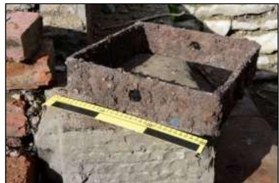
Photo 14 – Close-up of metal band found fitted to the rods above the East Flue.
