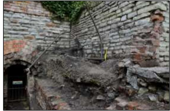
Photo 12 – Cleared area above East Flue. Both metal rods were threaded through a 'square' band, seen in close-up in photo 14.
