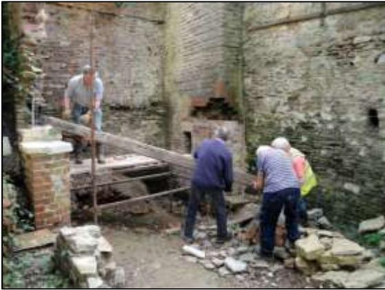
Photo 9 – Manhandling the bracing beam into place in the Old Boiler House.
