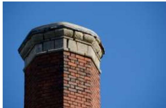
Photo 2 – ...the top with the reinforcing concrete ring in place in February 2015, but before repointing started...
