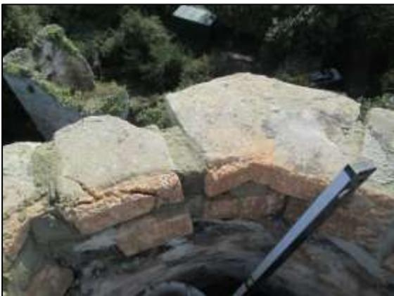
Photo 5 – Rebuilding the top of the chimney. © C Skelton, 2014.
