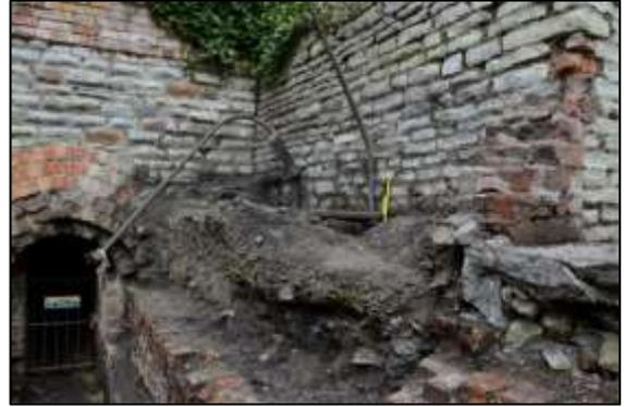
Photo 12 – Cleared area above East Flue. Both metal rods were threaded through a 'square' band, seen in close-up in photo 14.
