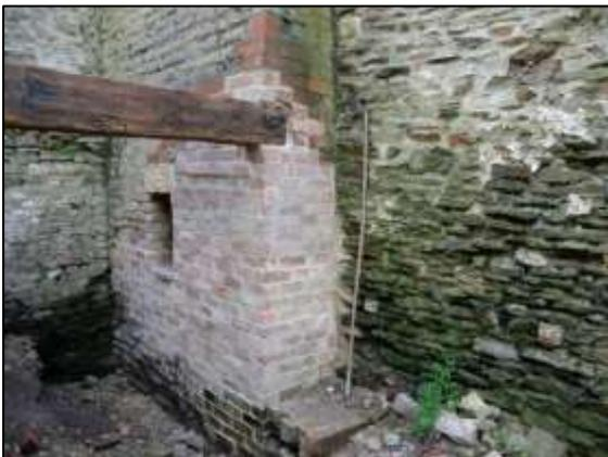
Photo 10 – The finished rebuild of the base of the chimney, with the bracing beam in place.
