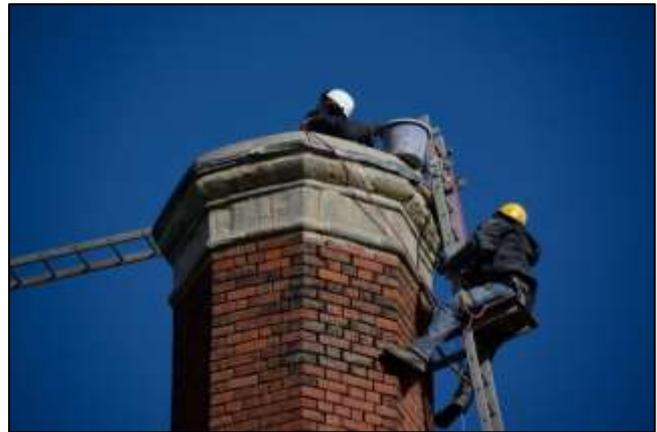
taken by the mason, C Skelton, in November 2014, show various stages in the rebuilding of the top and the casting of the concrete reinforcing ring. As is always the case with Brandy Bottom, another job surfaces as soon as one is finished. The pointing of the brickwork at the top of the chimney appeared to be in good condition when viewed from the ground. That was not found to be the case on closer inspection, and the top 6 feet will have to be repointed at a later date.
