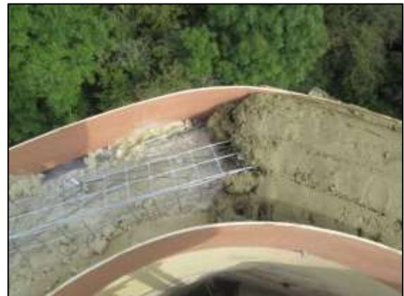
Photo 7 – Casting the concrete ring in situ. © C Skelton, 2014.
