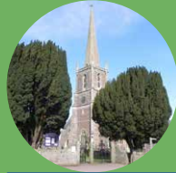
Winterbourne Parish Church
