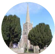
Winterbourne Parish Church
